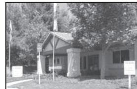
Creekside Senior Apartments
